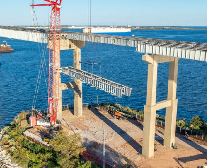
▲ The removal of the first steel girder on the south side of the bridge.
