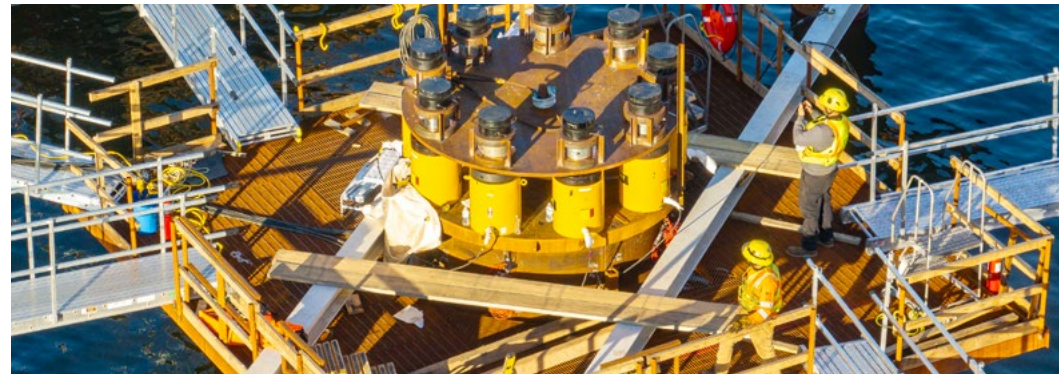
▲ Crew installing the jack system on a test pile.
