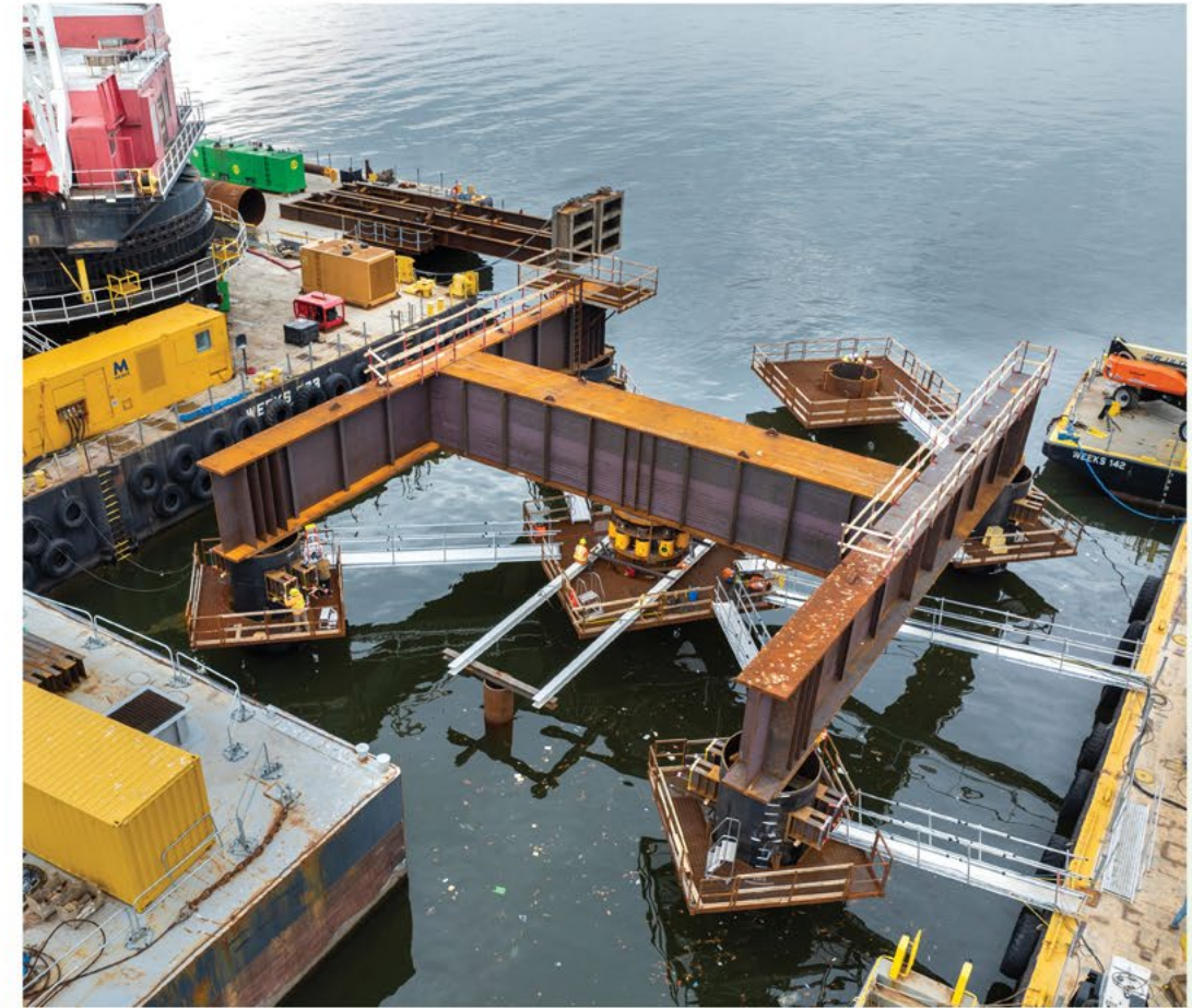
▲ The load frame placed on the test piles.
