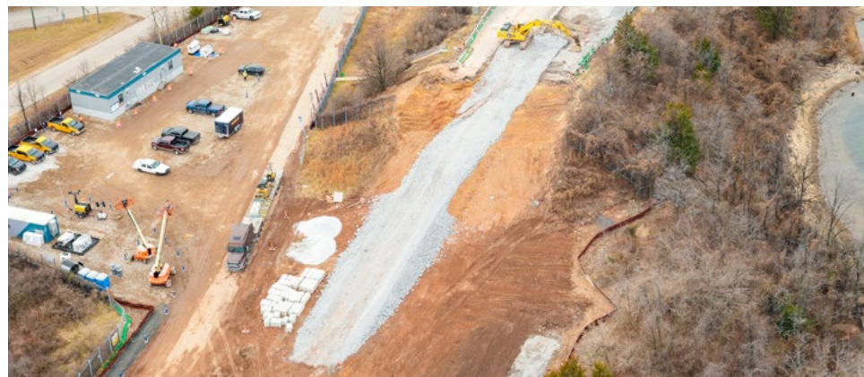
▲ Building temporary access roads.
