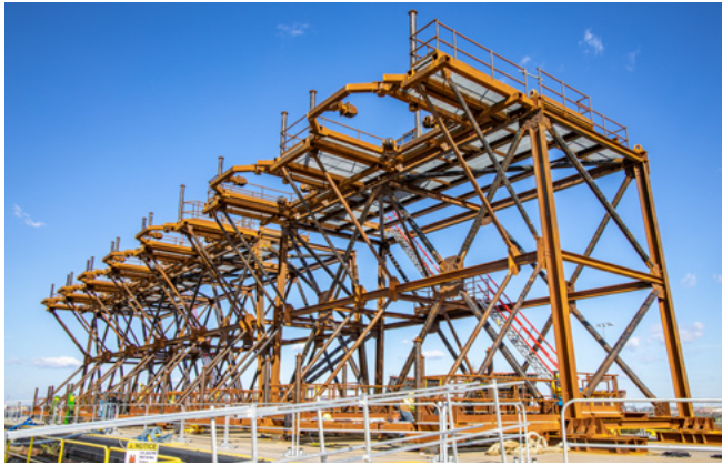
▲ Pile driving template.
