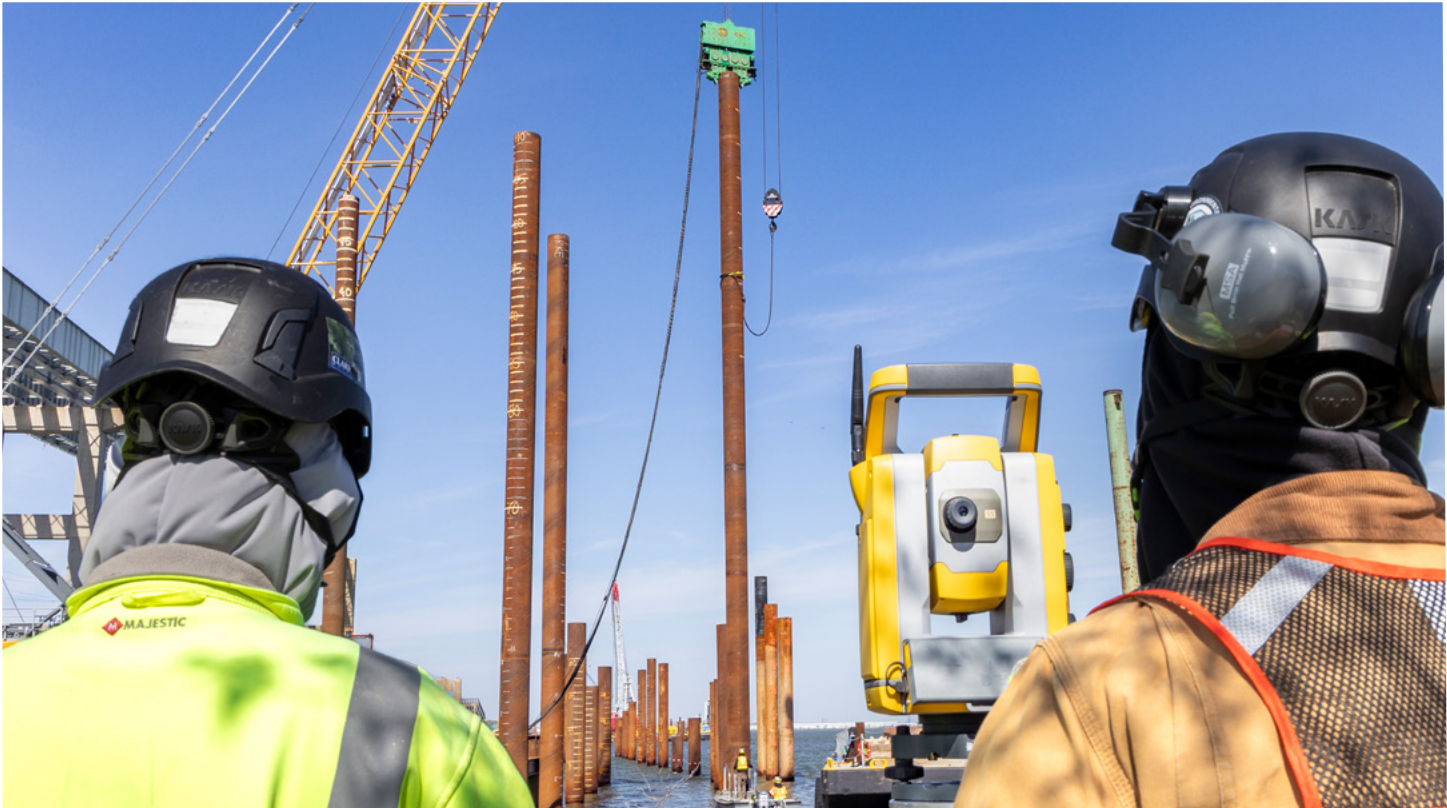
Surveyors on land use precision instruments to measure elevations, distances, and angles, helping to determine the exact locations where the crane will place the steel piles. ▲
