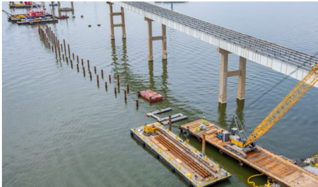
▲ Trestle construction on the north side.
