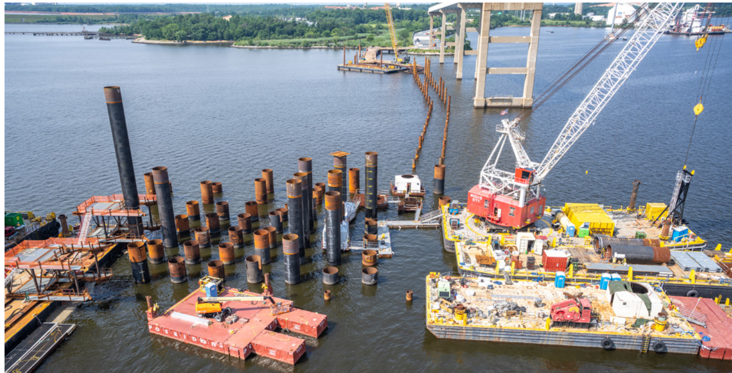
▼ Permanent foundation piles and pier protection piles at the south pylon (Pier 24).
