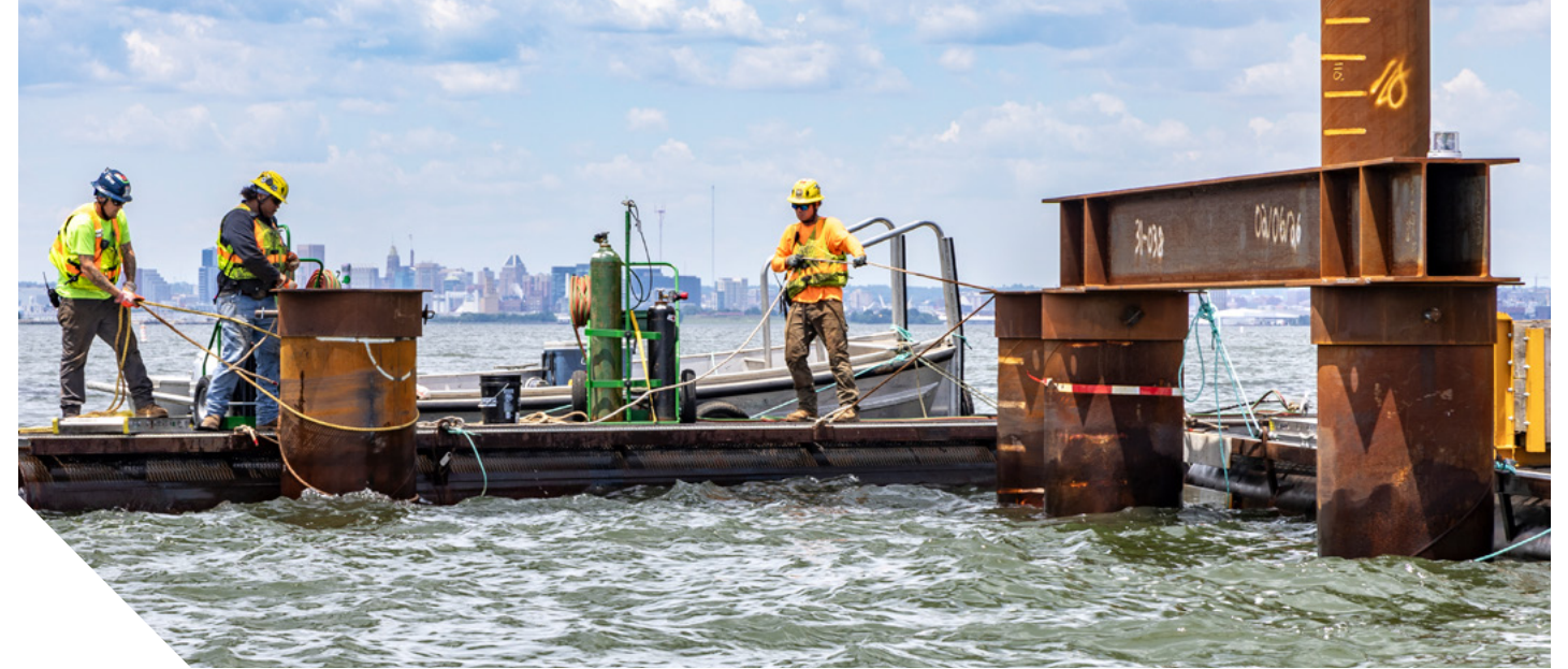
▲ Crews installing pile bonnets and cap beams for the trestle (work platform).
