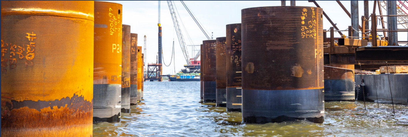
Permanent production piles in the foreground at the south pylon (Pier 24), with pile driving underway at the north pylon (Pier 25) in the background.
