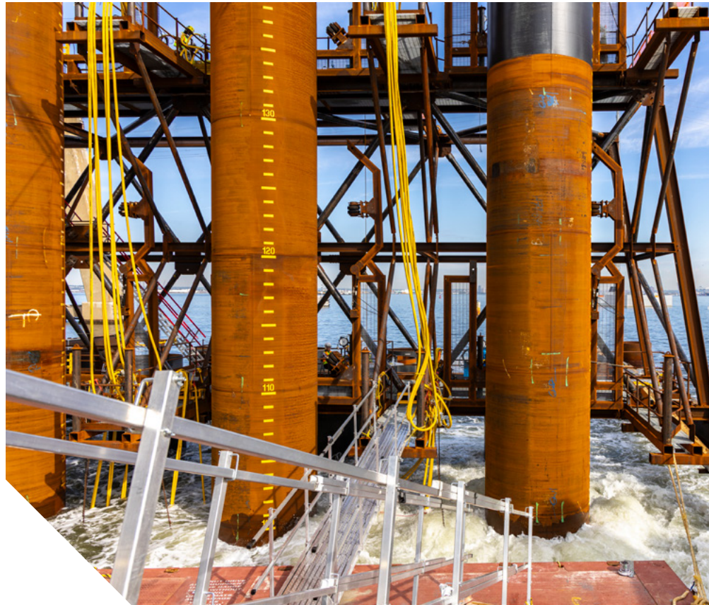
▲ The bubble curtain releasing compressed air around the pile being driven.
